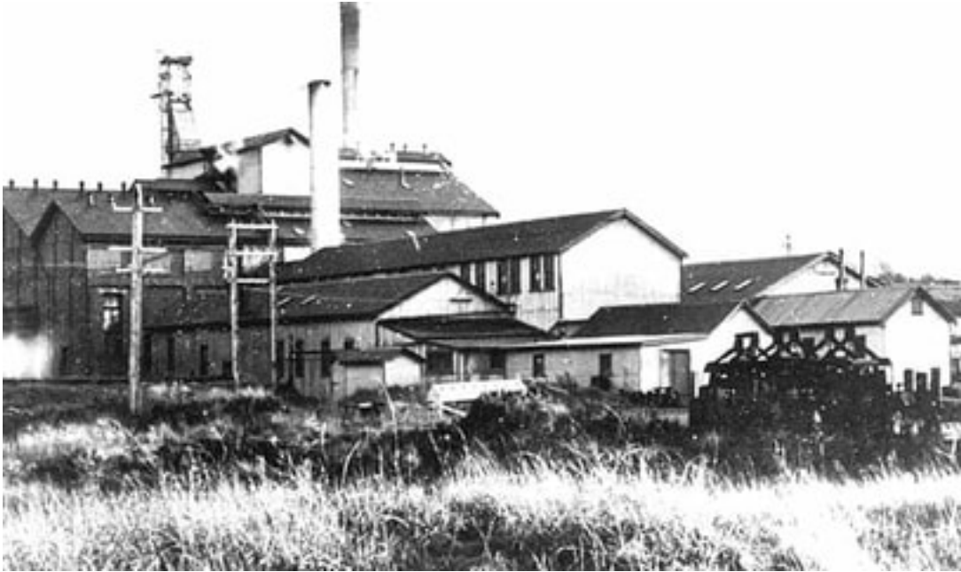
Wonthaggi Power Station powered the town from 1912 to 1966.
