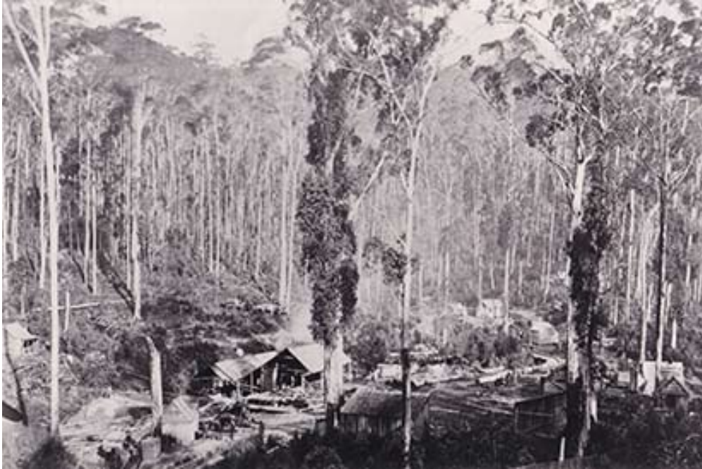
Original vegetation. The forest at Archies Creek before clearing the land for agriculture. This is Kennedy's Mill on Mill Rd. Archies Creek,
